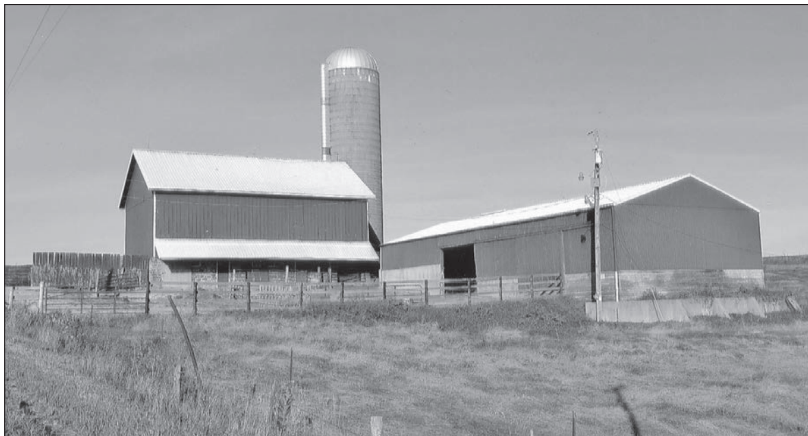
An early dairy barn constructed east of Monticello on County Highway C, still in use, but not for dairying.
