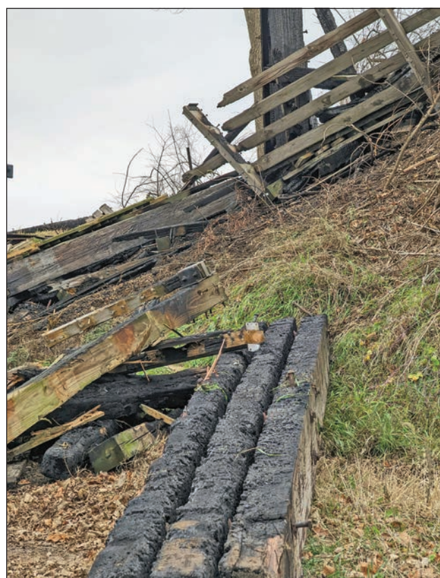
FRIENDS OF BADGER STATE TRAIL PHOTO Brodhead Independent Register Someone set fire Nov. 10 to a bicycle bridge on the Badger State Recreation Trail at Round Grove Road. Investigators are seeking tips through Green County Crime Stoppers.
