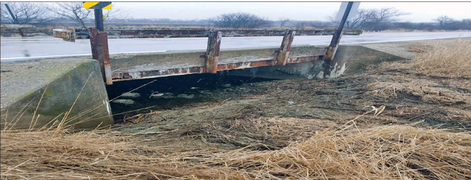
Right: The County Highway S bridge north of Highway 11 was replaced in 2022; it was flagged as unsafe and a weight limit was to be posted at 25 tons. This is an important route for both major cheese factories as well as large farming operations. Above: Of his crew, seen here grading for bridge replacement in the Town of Clarno, County Commissioner Chris Narveson said, "Green County Highway is blessed with one of the best groups of "can do" workers in the State. I am proud to be part of this innovative group."
