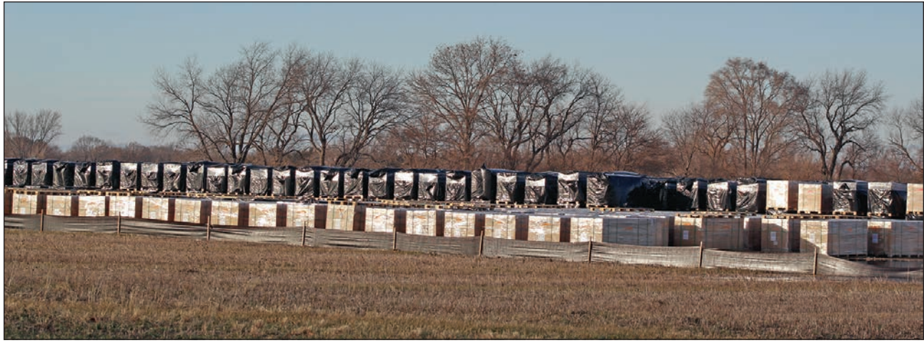
Solar panels and materials await construction in Alliant's Albany Solar Project, which is leasing about 400 acres in the Town of Decatur and Green County.
